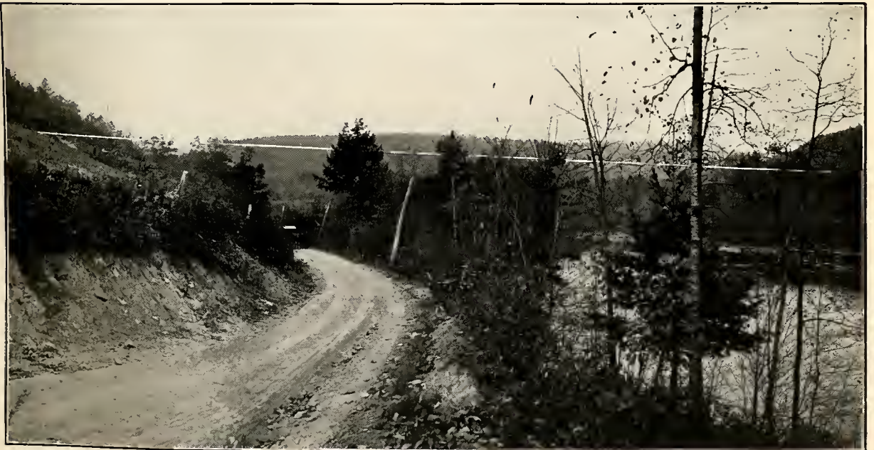
CLARION RIVER, PA., OCTOBER, 1910. View up stream, showing crest of proposed Dam No. 4.
